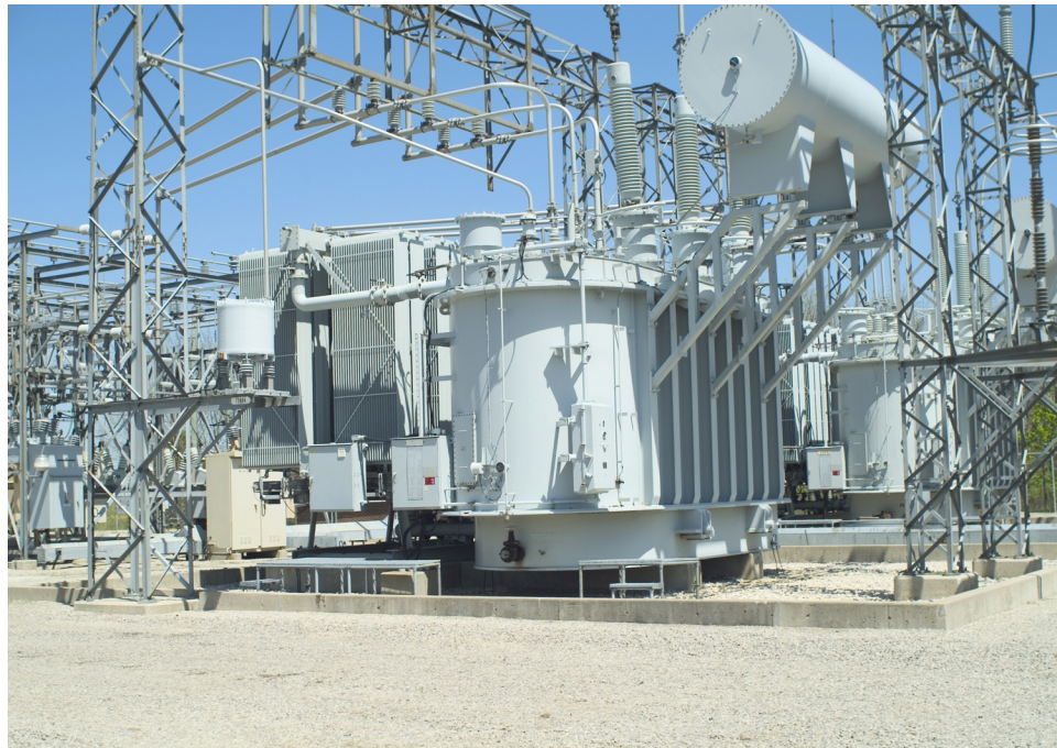
Three-phase transformer bank used for power distribution.
